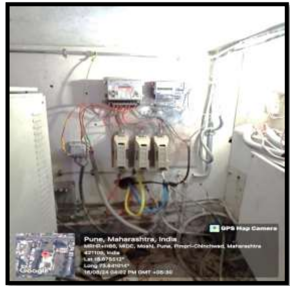
Wheeling to the grid
